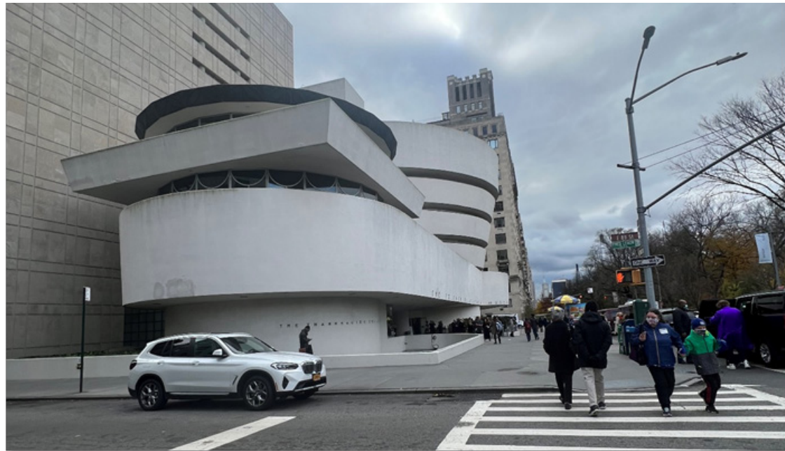
Fig 3 Guggenheim Museum (1959, New York), located at the intersection of naturalistic Central Park and urbanistic Fifth Avenue architecturally commands its context. Source: Photograph by author
